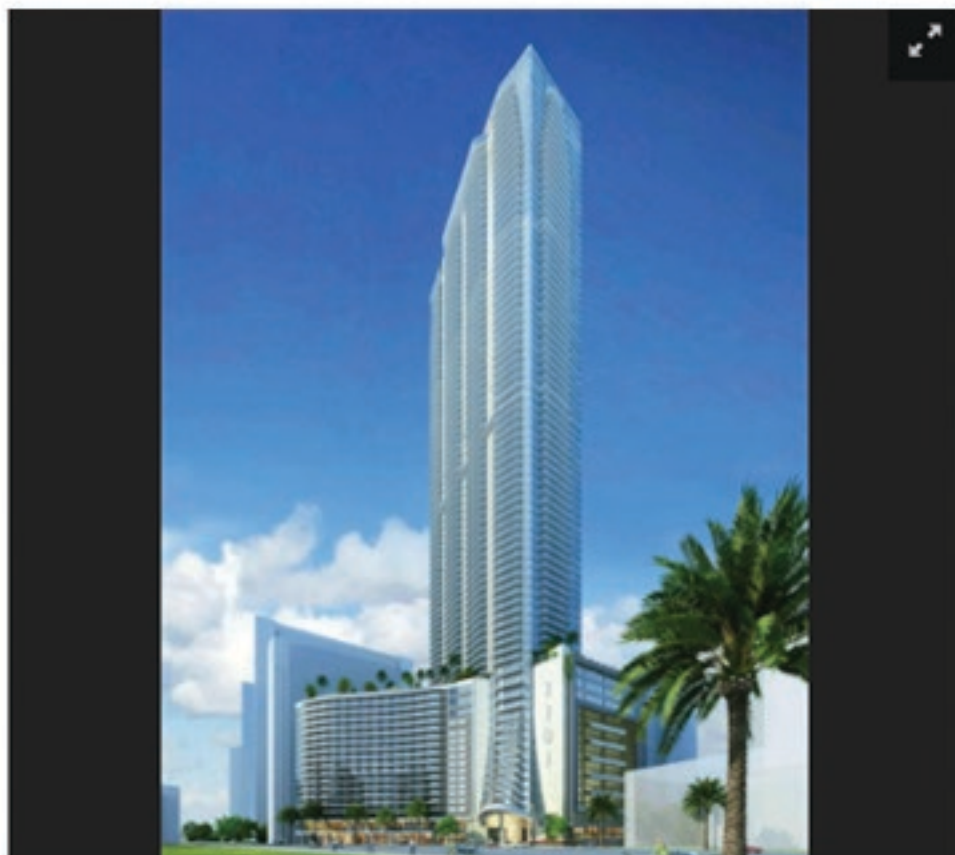
Panorama Tower in Miami will get a $4.5 million network from Atlantic Broadband.
